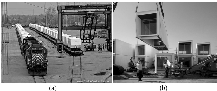
Fig. 1. Ready-made units: (a) temporary housing units ready to be transported (source: www.katrinadestruction.com ), and (b) local assembly of units. Source: http://exc.ysmr.com .
