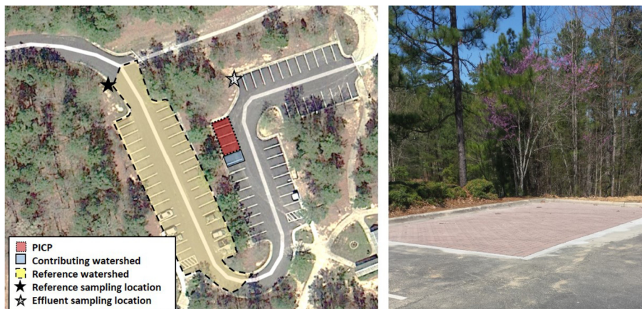
Fig. 2. From left to right: (a) aerial view of Piney Wood park: 50 m 2 of PICP (in red), 15.2 m 2 of contributing watershed area (in blue) and 1390 m 2 reference watershed (in yellow) with reference sampling location (black star) and effluent sampling location (white star); (b) Piney Wood PICP retrofit. (For interpretation of the references to colour in this figure legend, the reader is referred to the web version of this article.)
