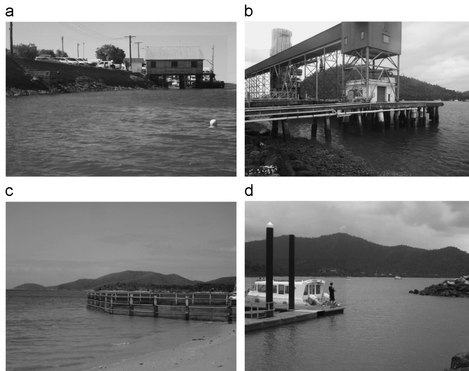
Fig. 1. Example of the engineering features in the Great Barrier Reef heritage estate. (a) rock wall for foreshore stability and protection in Townsville; (b) coastal port facility in Gladstone; (c) swimming netting area near Bowen; and (d) pontoons and boat ramp, with a recreational angler using this feature near Cairns. See Fig. 2 for township locations.
