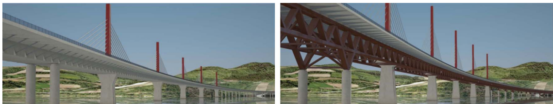
Fig. 1. Concrete bridge (left) and timber bridge (right) designs for the new Mjøsa Bridge (Statens Vegvesen, 2015).
