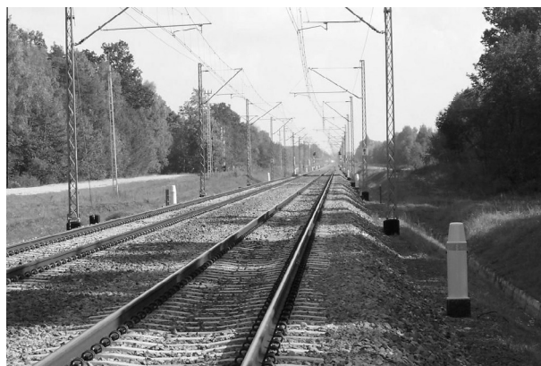
Fig. 1. Installation of UOZ-1 protective devices along the railway line.
