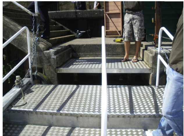
Fig. 1. Steps and landing platform.
