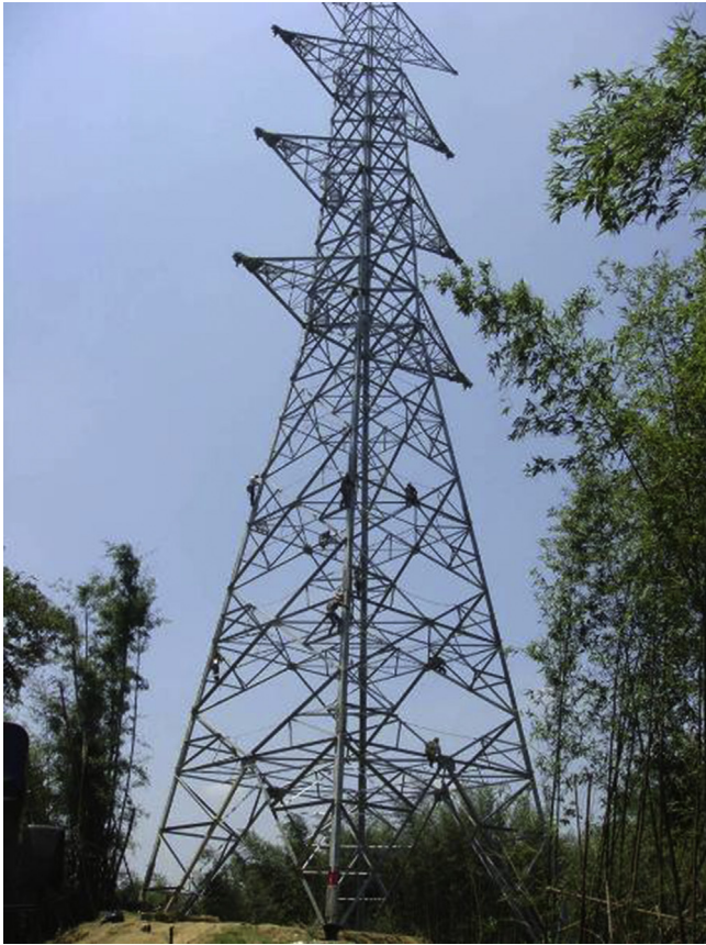
Fig. 1. The primary structure of a high-voltage transmission tower with a height of 62 m.
