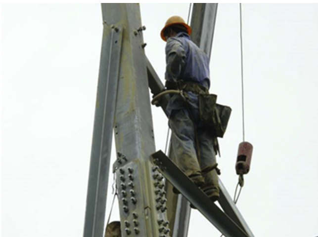
Fig. 2. The workspace of high-voltage transmission tower construction operations.
