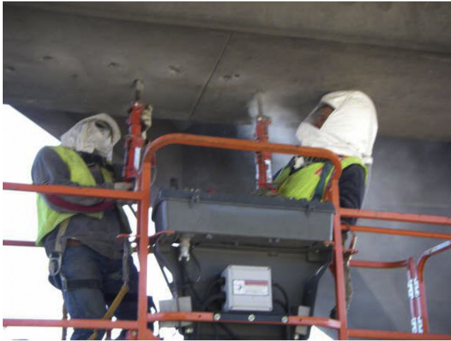
Fig. 1. Manual drilling with pneumatic rock drill for structural work.
