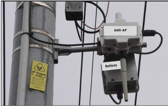
Fig. 1. Access point with backup SLA battery on a distribution line.
