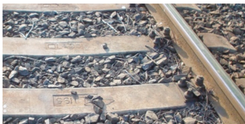
Fig. 1. Fouled ballast.
