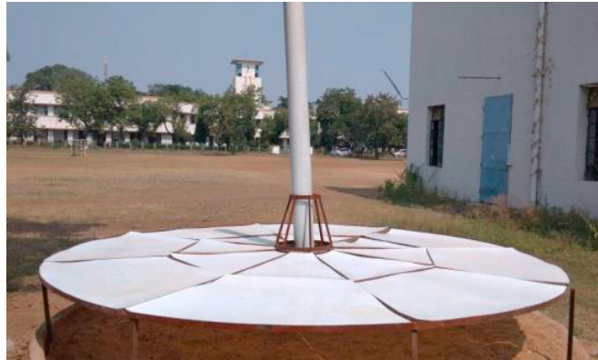
Fig. 1. Experimental setup of Solar Chimney Plant
