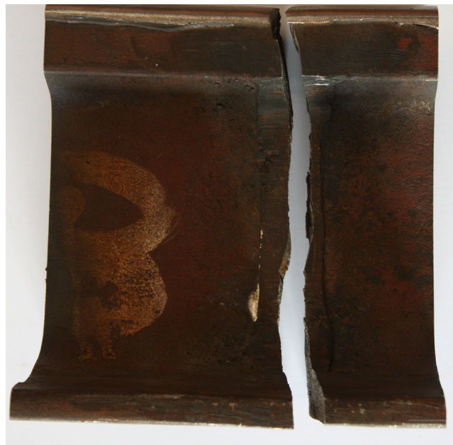
Fig. 1. Rail fracture position and crack propagation shape.
