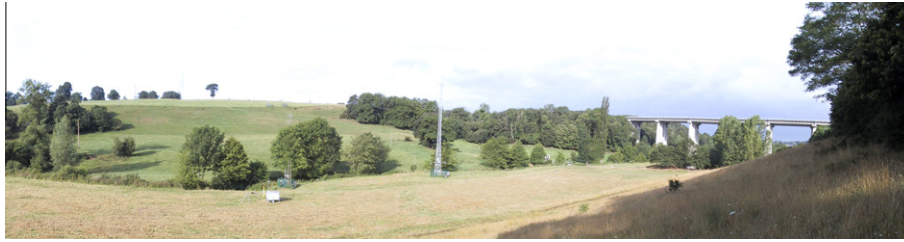
Fig. 1. LTMS – general view (looking northeast to southwest).
