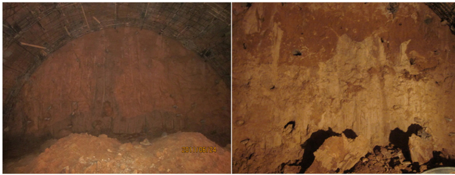
Fig. 1. Geo-condition in the section of collapse (tunnel face).
