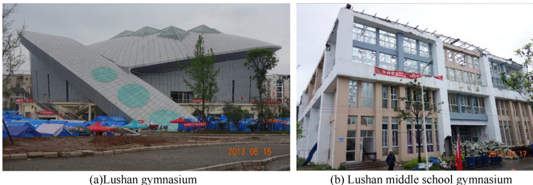
Fig. 1. Appearance of Lushan gymnasium and Lushan middle school gymnasium after the earthquake. (a) Lushan gymnasium. (b) Lushan middle school gymnasium.
