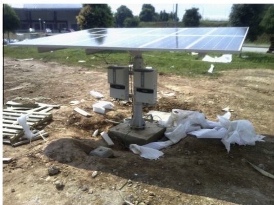
Fig. 1a. Installed fixed flat PV system.
