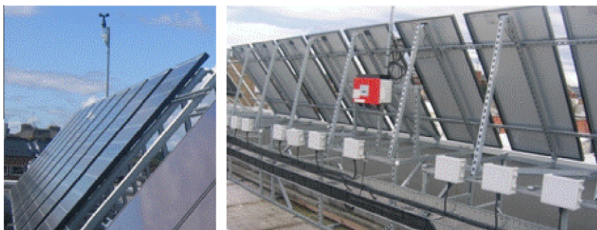
Fig. 1. The PV system installation.
