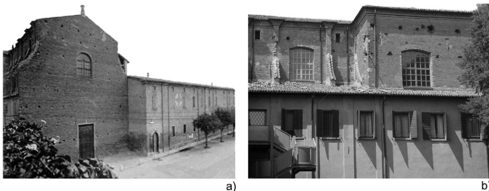
Fig. 1. Church of Gesù, view of the façade and annex (a) and of the south side with the lower annex (b).
