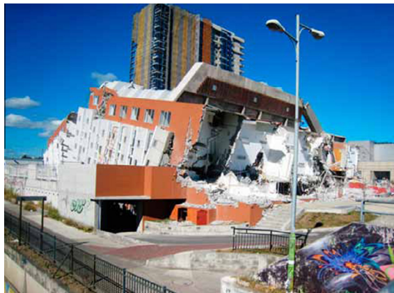
Fig. 2. Collapsed Alto Río tower, conception, Chile, 2010 [2].
