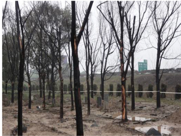
Fig. 2. The fired trees around fracture pipeline.
