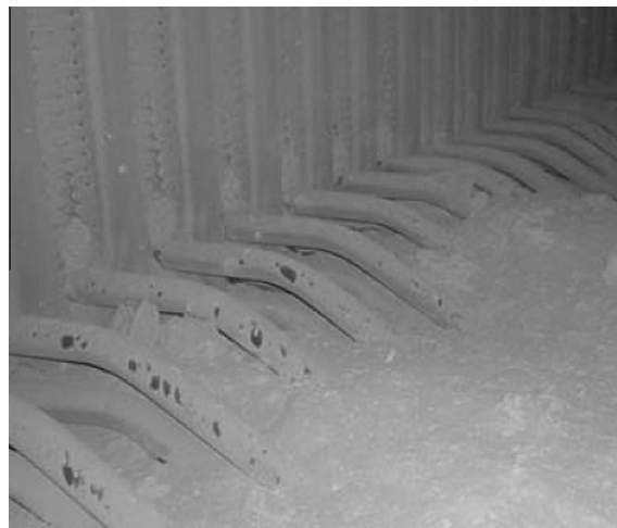
Fig. 1. Massive clinkers covering superheater region.
