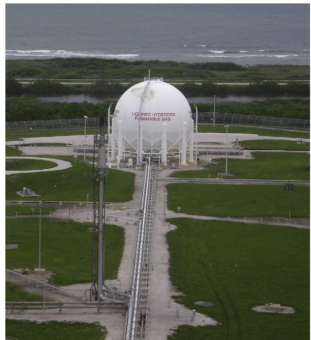
Fig. 1 – Liquid hydrogen is carried to the launch pad through a cross country line from an 850,000 gallon (3,200,000 L) storage tank. The vertical column is the flare stack where hydrogen boil-off is burned. The Atlantic Ocean is in the background.
