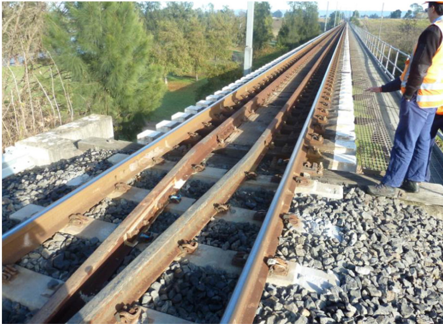
Fig. 1. Ageing railway transom bridge.
