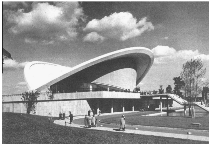
Fig. 1. Original structure of the congress hall before sudden collapse, photograph in 1960 [3].
