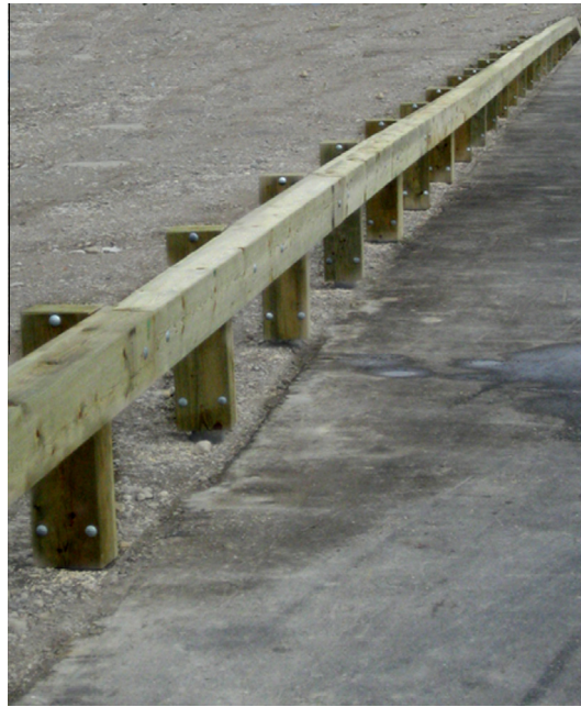
Fig. 1. Steel reinforced wooden road safety barrier.
