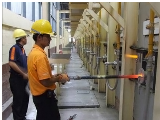
Fig. 1. The appearance of pipe during operation.
