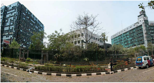
Fig. 1. Blast damage to glass facades on buildings adjacent to the Australian Embassy in Jakarta, Indonesia, 2004 (image used with permission of the Australian Federal Police).
