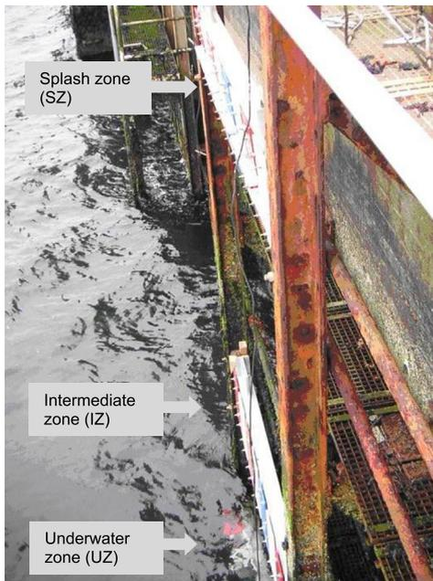
**Fig. 1.** Corrosion zones on offshore wind power structures, and sample exposure at the test site at Helgoland.
