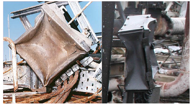
Fig. 2. Two typical damaged boxes (Courtesy of the Health and Safety Laboratory).
