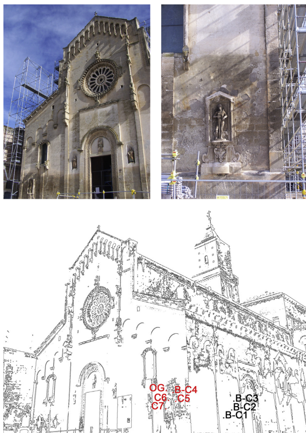
Fig. 1. Facade of Matera Cathedral (Matera, Italy) with the dark alteration in the lower part of the structure (up to 6–8 m) and details of the niche with St. Eustache statue (above). The provenance of the samples (bottom).
