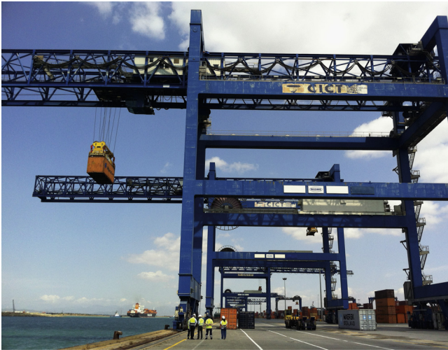
Fig. 1. The quayside container crane at the Cagliari International Container Terminal (CICT) in Cagliari (Sardinia, Italy).
