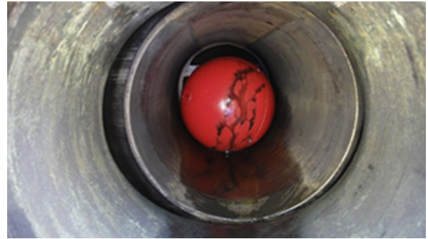
Fig. 2. Detector inside the pipeline launcher.
