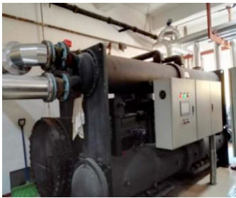
Fig.1 Sewage source heat pump heat pump
