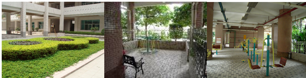
Fig. 1. Building piloti design in Guangzhou, China.
