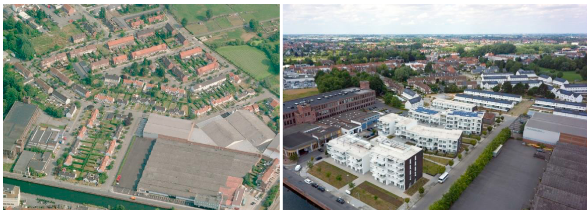
Fig. 1. Aerial view of the original (left) and transformed (right) Venning district.
