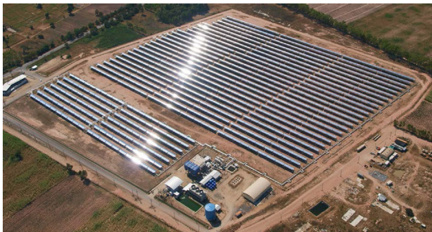
Fig. 1. Aerial view of TSE1, Kanchanaburi, Thailand. Source: Solarlite.
