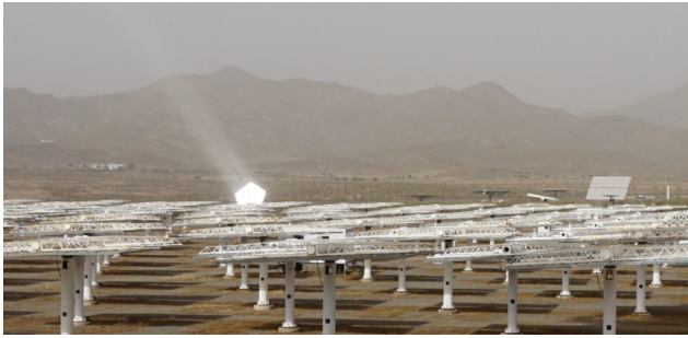
Fig. 1. Low visibility and substantial light scattered by large particles in the atmosphere at PSA on 2016-02-22 at 14:30 local time. Solar radiation reflected by the heliostats is visibly attenuated by scattering.
