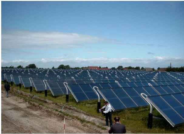
Fig. 1. Solar collector field with a high number of rows with flat plate collectors.
