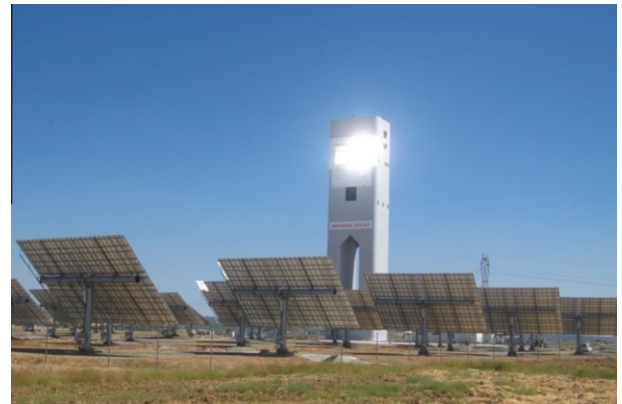
Fig. 2. Solugas plant operating.
