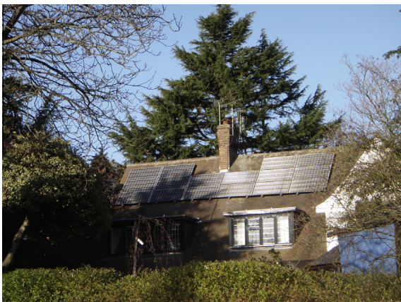
Fig. 1. Photograph showing a south facing PV-system which is not heavily shaded but the energy yield loss due cell mismatch is significant.
