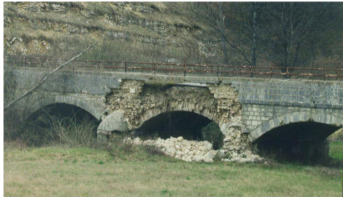
Fig. 2. Damage of a masonry bridge [3].
