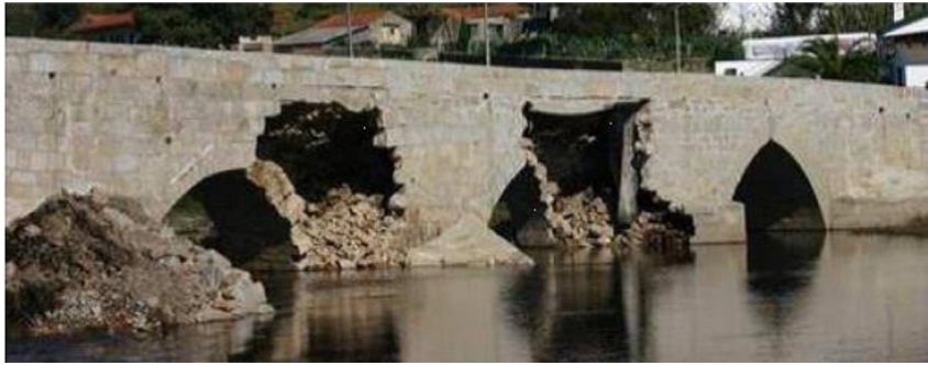
Fig. 1. Upstream view of collapsed arches and piers [1].
