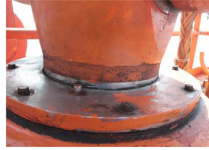
(b) The damage position of right mooring leg
