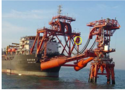
(a) Damage has occurred, but it is still in service
