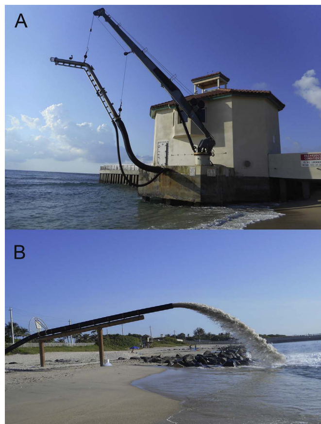
Fig. 2. Photographs taken of the South Lake Worth Sand Transfer Plant system in June 2016. A) sand transfer plant on the north jetty to the South Lake Worth Inlet. B) outflow pipe along the eroded beach just beyond the south end of the South Lake Worth Inlet.
