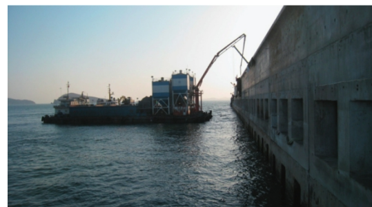
Fig.2 The perforated breakwater with five perforated walls built for Dalian chemical production terminal, China.
