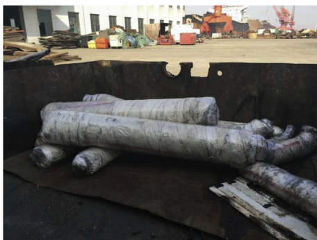
Fig. 4. The pipes containing asbestos.
