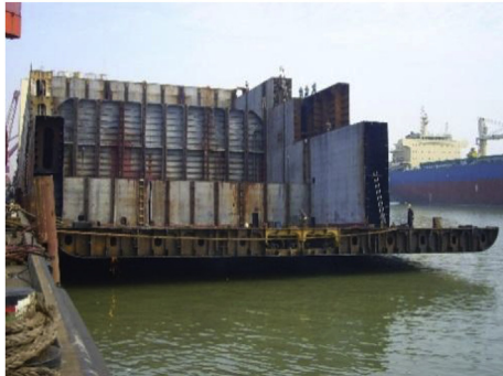
Fig. 2. Dock shipbreaking method pollutes the environment less.
