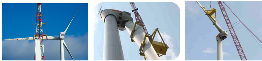
(a) Horizontal mounting (Siemens, 2014b) (b) Vertical mounting (Liftra, 2012) (c) Inclined mounting (Liftra, 2012)
