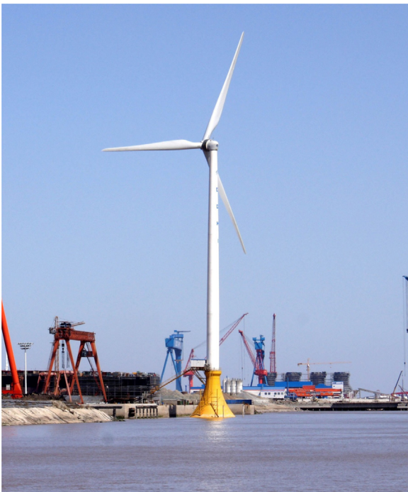
Fig. 1. The 2.5 MW offshore wind turbine supported by CBF.
