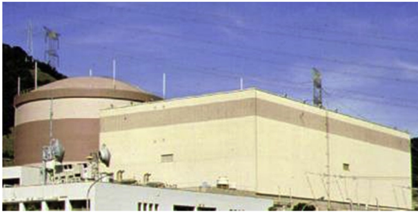
Fig. 1. Tsuruga Nuclear Power Station unit 1. Turbine Building: the square building in the right. Reactor Building: Cylindrical building in the back-left side.
