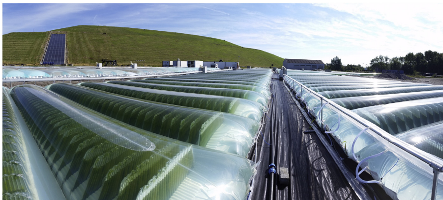
Fig. 1. View of a ProviAPT™ microalgae production plant of 48 m 3 culture volume.
