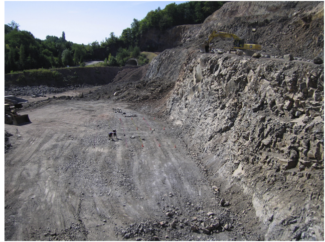
Fig. 3. Rock fall drop tests in progress at the Klösch Quarry in Austria.
